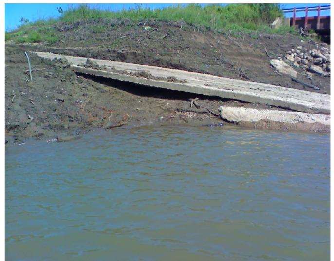
*Flood damage to Ladd Bridge boat ramp.*
