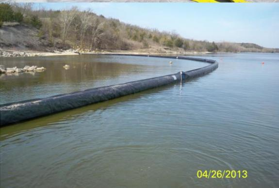
The fish barrier has worked very well so far this year and anglers have done a good job of not tampering with it. The barrier will be removed for cleaning and repairs as soon as the irrigation season is complete, and will be stored until next year. Hopefully, anglers will reap the benefits with improved fishing in the next few years.
