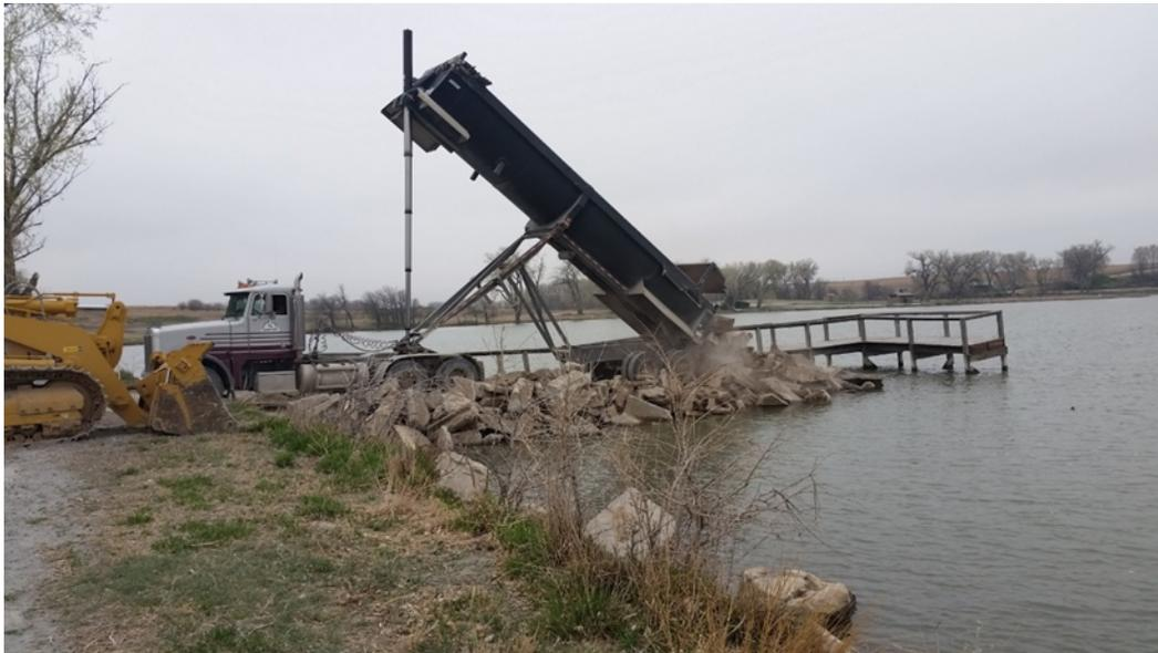
*Placing broken concrete to construct a fishing pier, note the old wooden dock in the background*
