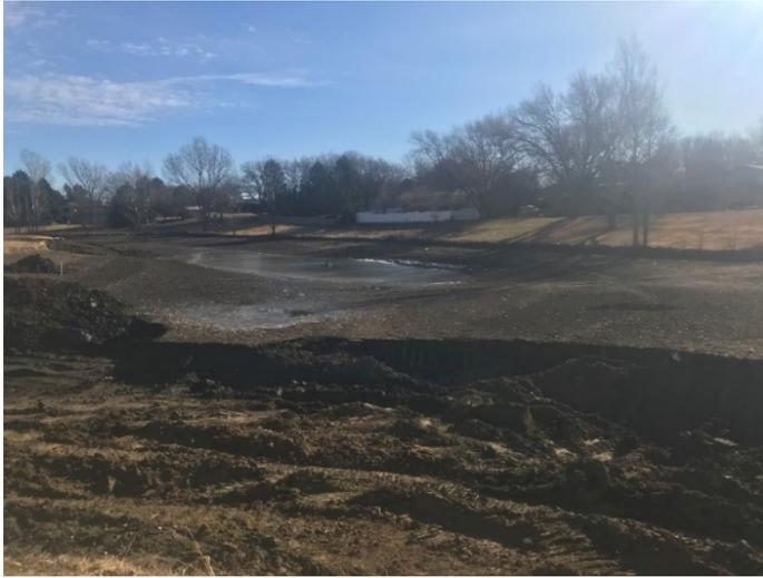
*Early stages of excavation at Villa High, note sediment thickness and overall shallowness of basin*
