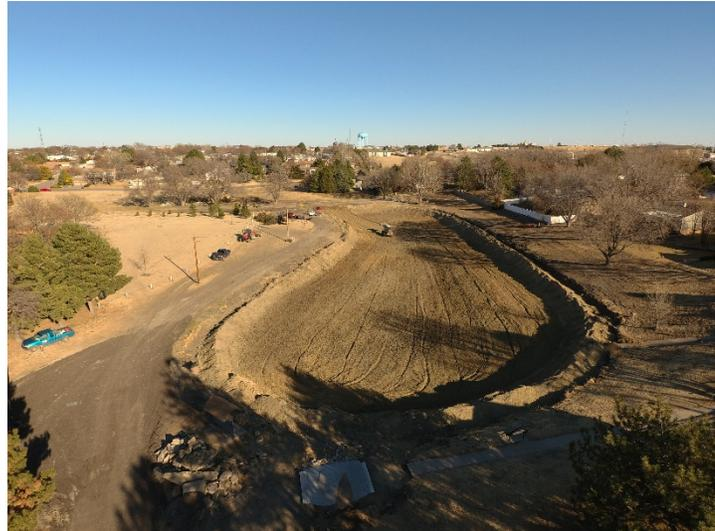
*City and county staff drying and stockpiling bottom material prior to basing sealing*
